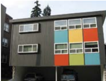
The Jan Tun Apartments reduced water use by 25% by replacing toilets in 14 units.
