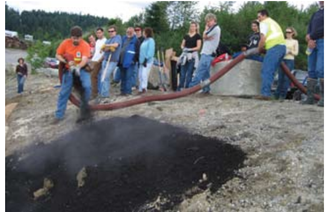
Contractors learn how to install a compost blanket, to promote successful plant establishment on hillsides with poor soils and no irrigation.
